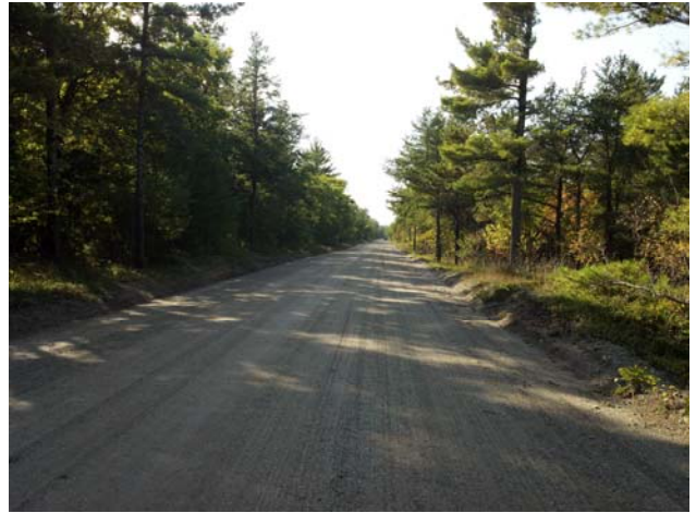
Segment 1: Lake Michigan Drive and picnic facilities
