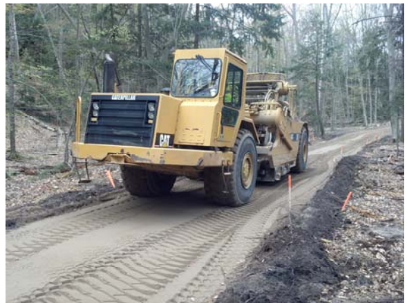
Grade Excavation of 60' Dunes
