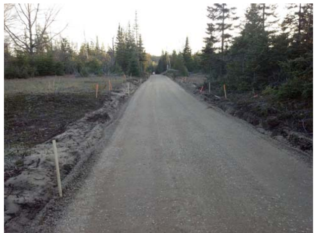
Trail construction that would be typical of “Along the Shore” route
