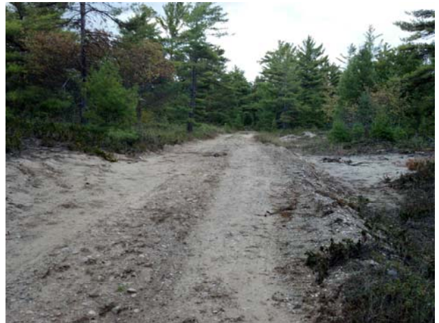
Segment 3: Uses existing Juniper Lane – a gravel roadbed
